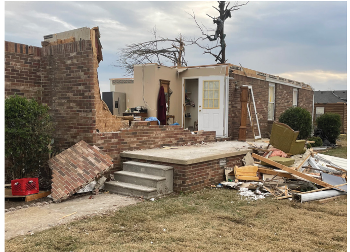
The House in a Box program will help many families in Kentucky and Tennessee obtain essential household items to make their rebuilt homes livable. The photo above shows a Tennessee home that was destroyed by the tornadoes. Photo by American Red Cross
